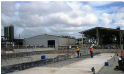
Earlier this year Rocla was awarded a significant contract to provide pre-stressed concrete decking for the upgrade to the Hay Point coal terminal in Queensland. During the 16-month long project, Rocla will supply main contractor, Bechtel, with 2,000 pre-stressed concrete decks, each measuring between seven and 24 metres in length.
