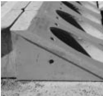
Low-profile sloping face headwall
