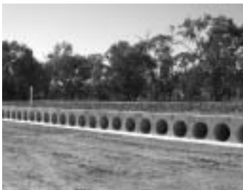
25-cell 750mm diameter pipe headwalls under rail line
