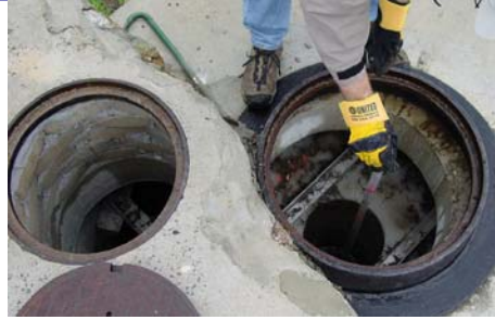
Figure 4 – Checking Sediment using a Probe
