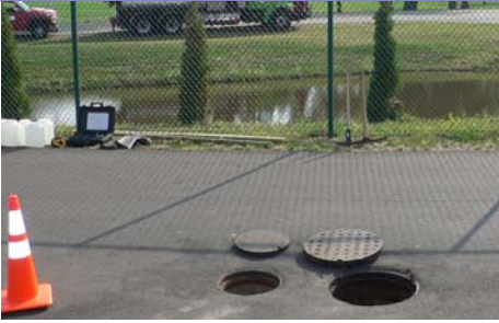
Figure 3 – Inspection and Maintenance Covers
