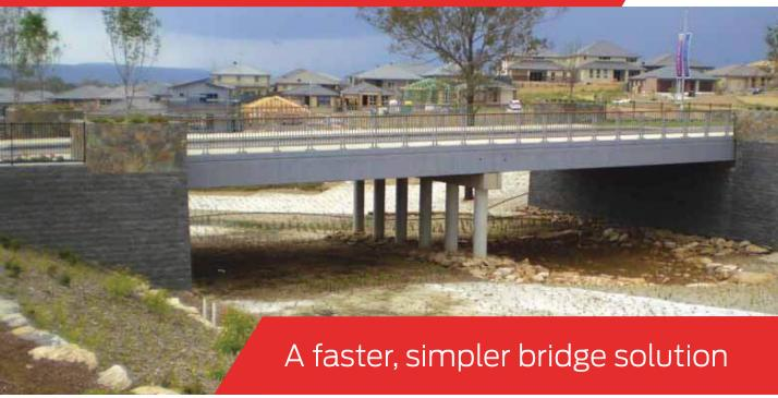
Rocla's fast and simple-to-construct M-Lock Bridge System was used to deliver a 30 metre long, 14.6 metre wide crossing over a natural water course at the Mulgoa Rise subdivision, near Penrith.
