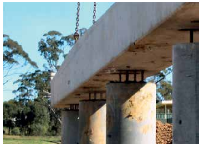
FIG. 4: PLACING PRECAST HEADSTOCK
