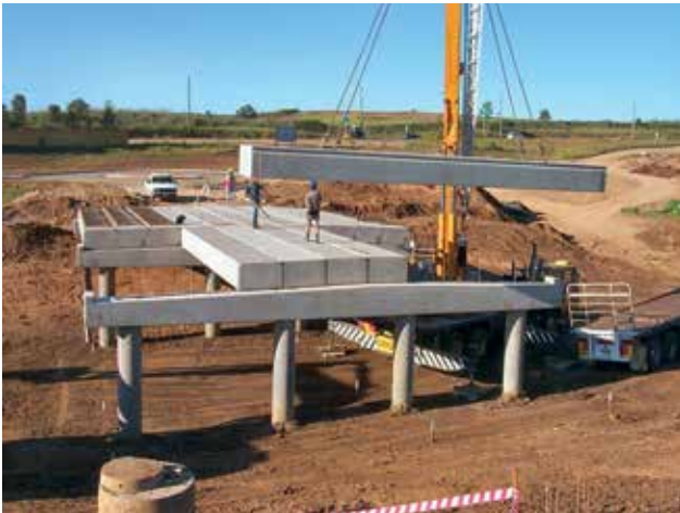
FIG. 5: INSTALLING PRECAST PLANKS
